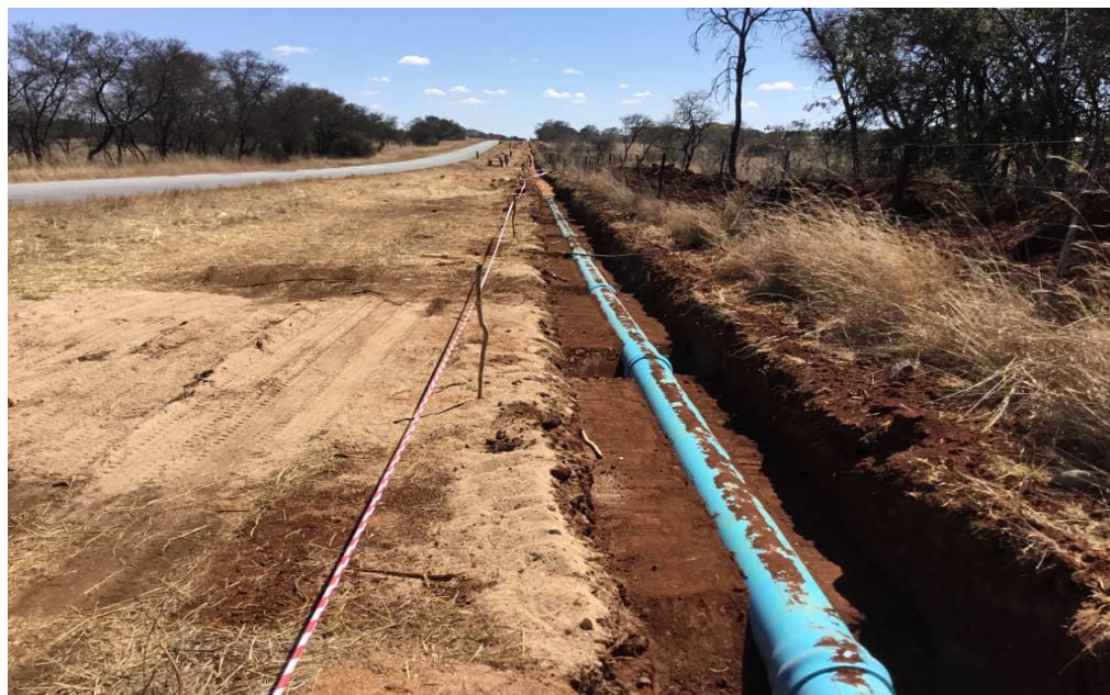
Pipeline conveyancing from Chivhu dam project to Chivhu town
