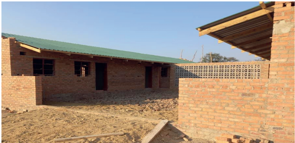
Umgula Clinic under construction, Matopo RDC
