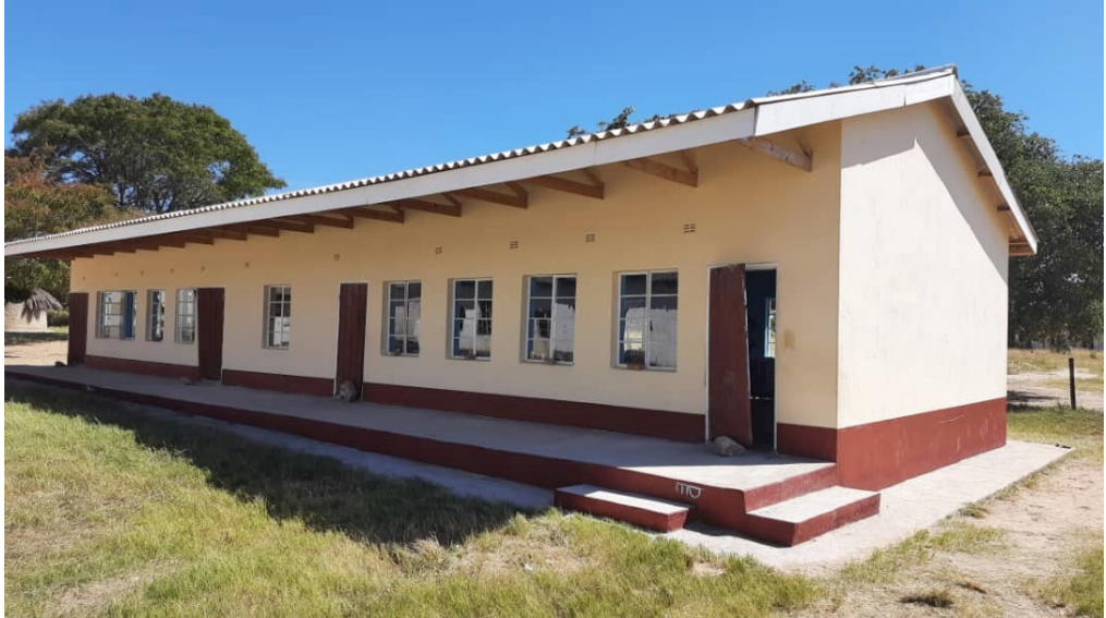
Completed Madzorera Classroom Block, Zvimba RDC
