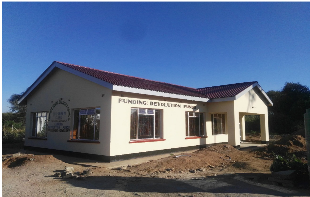
Chipangayi Clinic, completed staff house, Chipinge RDC
